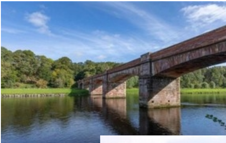
left - Mertoun Bridge below - view from the balcony.
